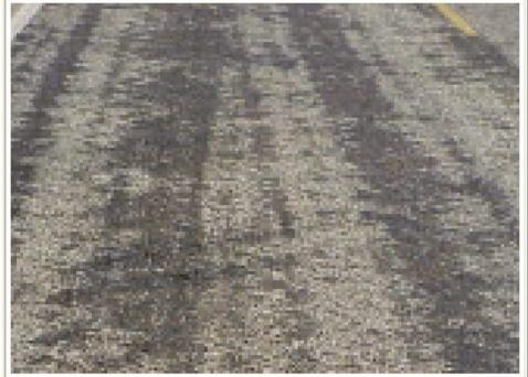
Loose materials (usually aggregate) that "ravel" from the surface or edges of the pavement, resulting in depressions which may fill with moisture and loose aggregate which may pose problems.
