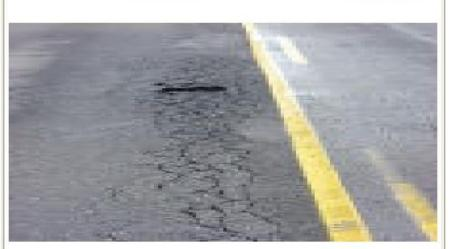
Is there anyone who doesn't know what a pothole is? They can be caused by a number of factors, but usually form when water gets into cracks and destroys the underlying structure. They most often appear when the pavement is most subjected to moisture -- in the early spring.
