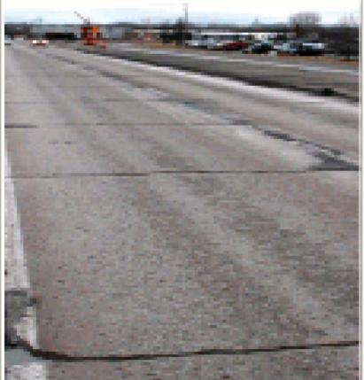
When a pavement cools quickly, it tries to contract. The internal stresses caused in this process may result in a series of cracks evenly spaced perpendicular (transverse) to the flow of traffic. There are two types of thermal cracks -- those occurring during a single falling temperature event, and those caused from damage accumulated after repeated temperature cycling.
