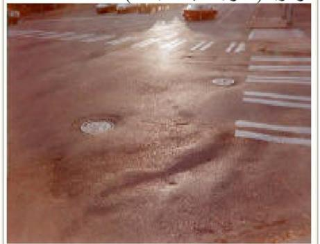
Pushing and Shoving: deformations of the pavement surface, most common in intersections, where there is braking and stopping traffic. It is easiest to detect at intersections where transverse striping becomes "wavy".
