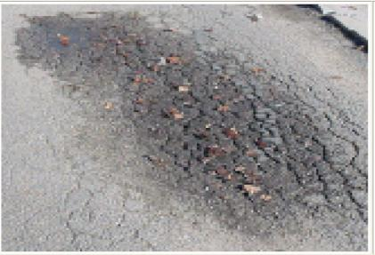
the liquid asphalt binder holds the pavement together and waterproofs the pavement. When moisture gets to the surface of the aggregate it can break the asphalt - aggregate bond, causing the pavement to disintegrate
